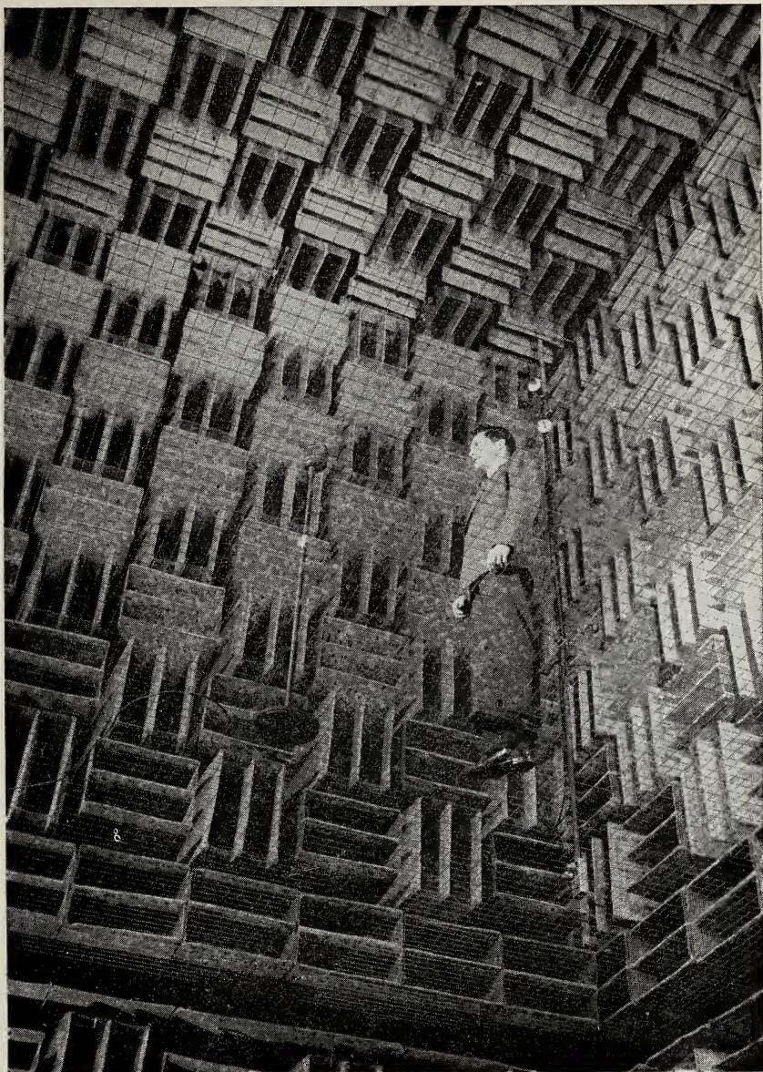
A modern anechoic room. ( Courtesy Bell Telephone Laboratories )
